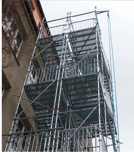
Whether it is a slim aluminium stairway, an extra-wide ascent for equipping the scaffolding or an approved emergency stairway tower – all the conventional options for changing levels can be implemented with RINGSCAFF ... and, of course, the "good old" ladder frame is still available as well.
