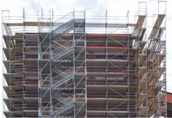
The concept of the Scafom-rux universal stair tower is based on a 12- to 24-leg scaffold base and meets the increased requirements resulting from the German Regulations on Places of Assembly.
