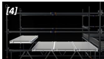
**[4]** The scaffold decks are then placed on the lattice girder.
