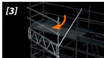
**[3]** Unfolding both lattice girders (right and left). Guardrails are attached for safety.
