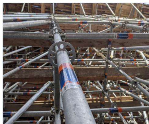
For the waffle slab construction of floors +2 and +4, large quantities of concrete had to be poured directly on site, each in sections of 16 by 16 metres. To make this possible, 130,000 m<sup>3</sup> of scaffolding was required to support the concrete floors at heights of up to 20 metres during the construction phase.
