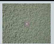
PU plugs - By insulating and sealing the anchorage point, the façade's thermal bridge is interrupted.
