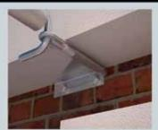
Variable - Thanks to the lengthadjustable ring bolt (threaded), the anchor can take-up insulation material thicknesses of 15 to 25 cm.
