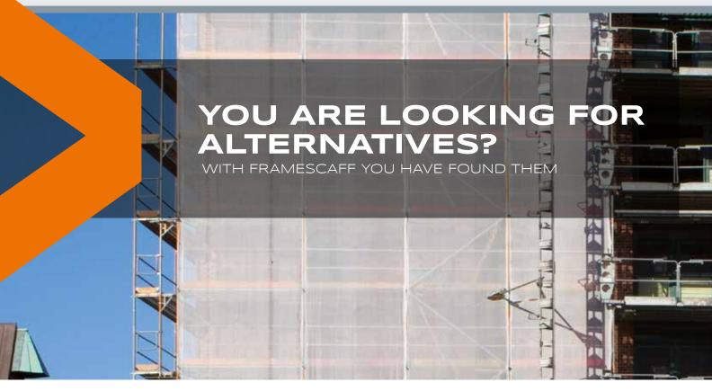
FRAMESCAFF is compatible with other, conventional façade scaffolding systems on the market with its standard width of 0.73 m and available lengths of 1.57 m/2.07 m/2.57 m and 3.07 m.
